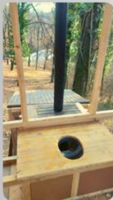
Compost toilet o toilette a secco
